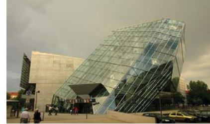
UFA Cinema Center http://openbuildings.com
