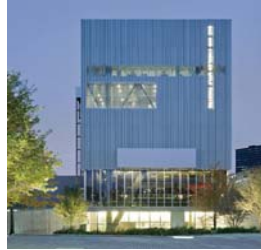
AT&T Performing Arts Center http://www.designboom.com
